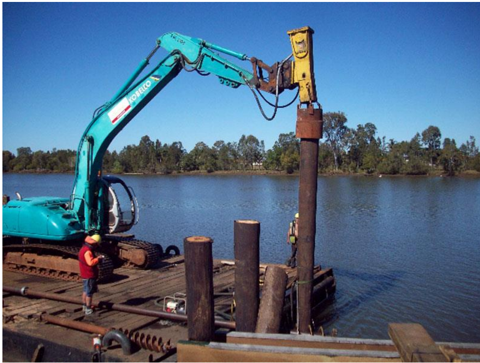
New piles being driven to extend infrastructure
