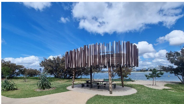
Figure 1 – Completed project- Moondarewa Spit Improvements
