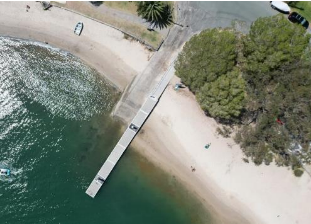
Murlong Crescent Boat Ramp, Tallebudgera
