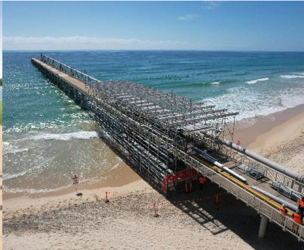
SBS Jetty Protective Coating
