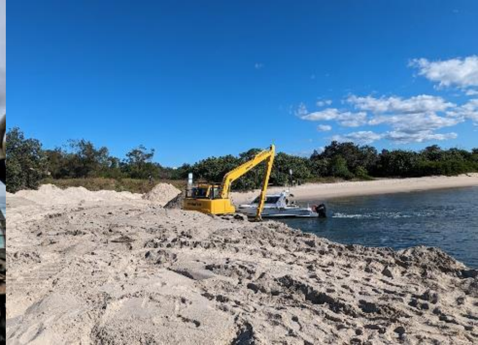
North Channel South Channel Dredging
